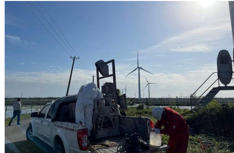
Suzhou Yaosheng Wind Field Inspection and Blade Maintenance Service Project
