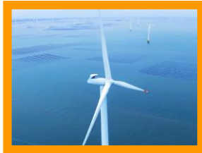
Offshore Wind Power
